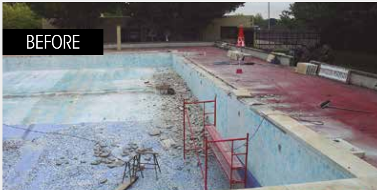
Cámping Ridaura (Llagostera - España). Renovating a skimmer pool to turn it into an infinity pool with Ergo S9 blocks.
